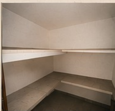
INTERIOR – SIDE VIEW
